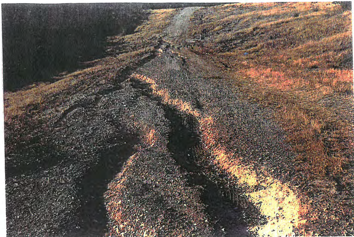
Photo No. 3: View of Travis County Landfill erosion of cover.
