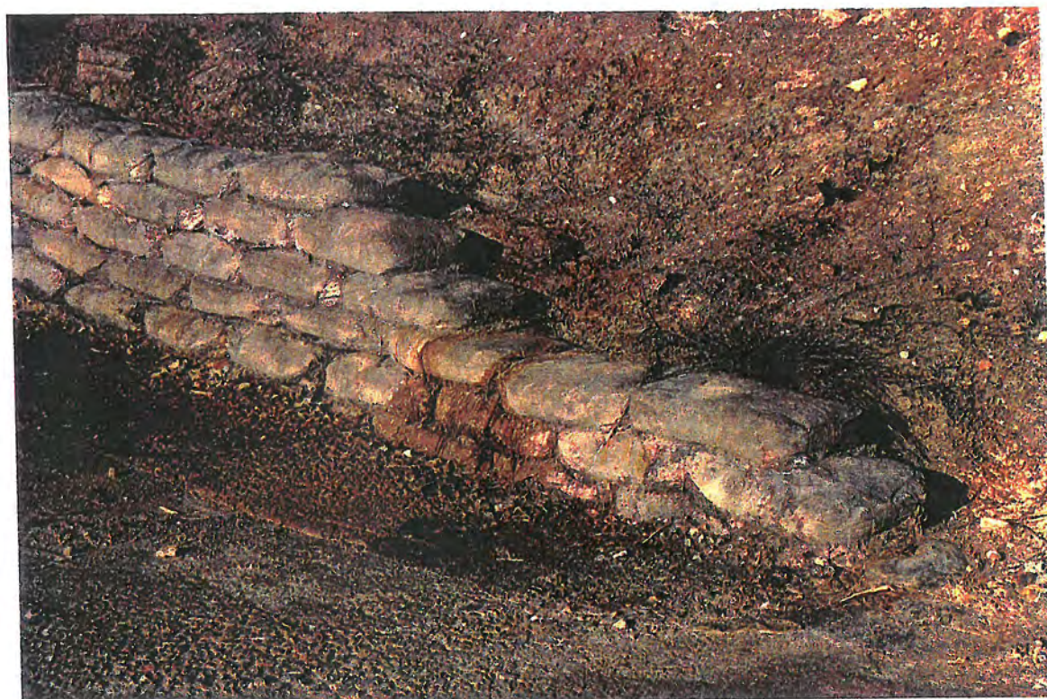
Photo No. 2: View of Travis County Landfill erosion of cover at leachate seep.
