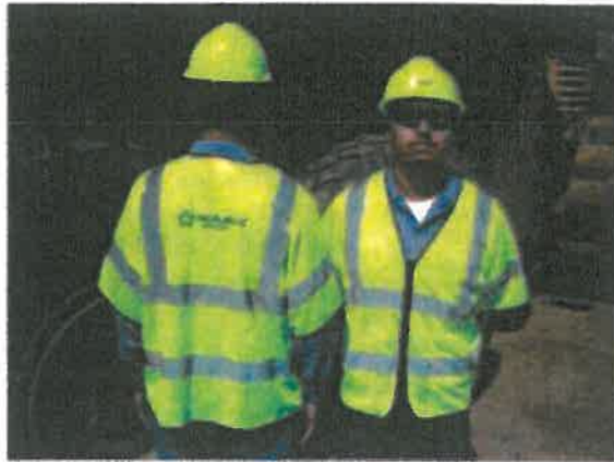
Always wear proper PPE at the working face.
